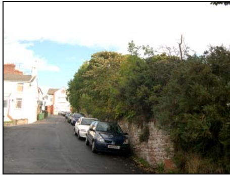
Fig.6. School Lane boundary
