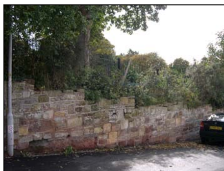
Fig.4. School Lane boundary
